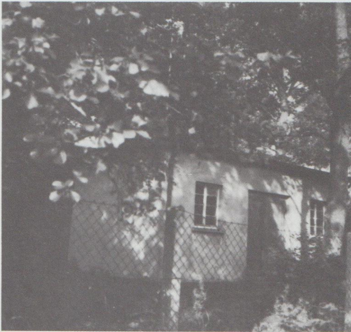
Pumpstation an den Quellen
