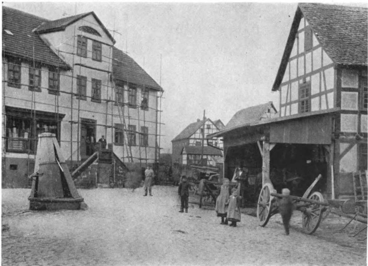
The town pump of Neustadt, which was the only source of supply before the water system was installed.
